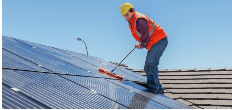
Fig 1.25: Picture of Cleaning PV panel
