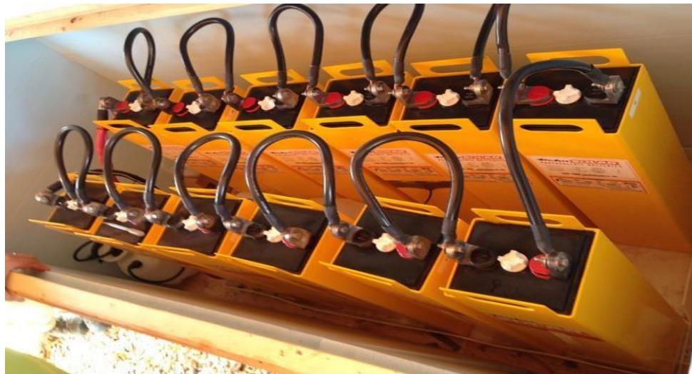
Figure 1.18: A bank of two strings of 2 volt batteries wired in series. Each string is 12 volts
